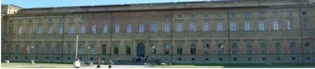
Figure 9. Northern façade of the Old Pinakothek
