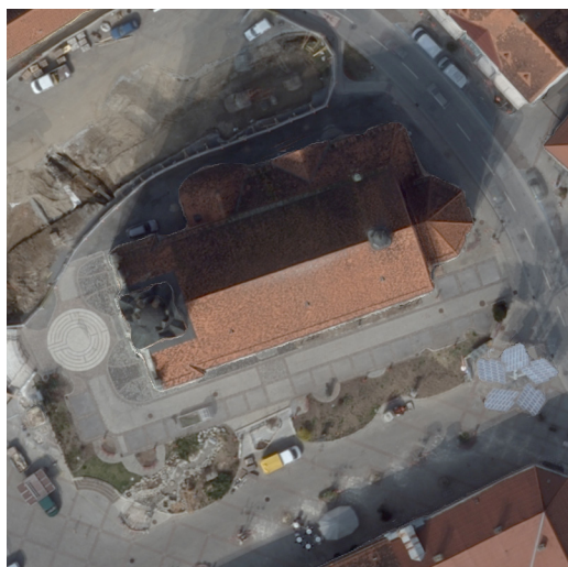
Fig. 9: Samples of a automatically processed orthoimage of the central area of Gleisdorf.
